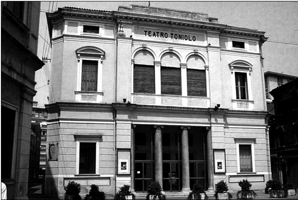
Fig. 3.33 Façade of Toniolo theater before works © Michielletto
