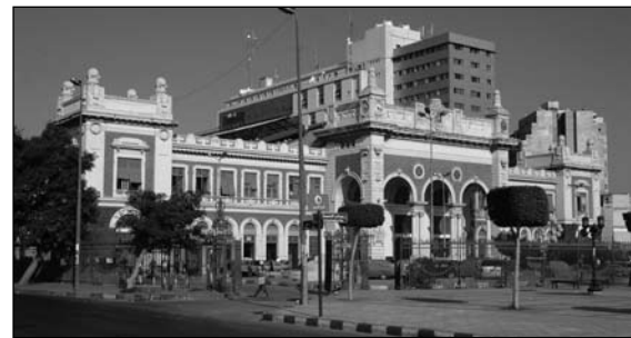
Fig. 3.13 Misr Station Square, a major transportation center. © AlexMed
