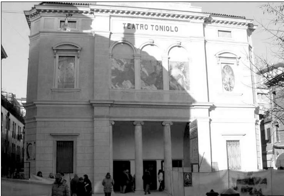
Fig. 3.34 Façade of Toniolo theater after works © Michielletto
