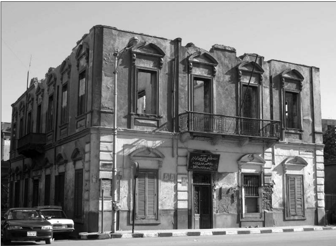
Fig. 2.48 The former Greek School and then the Greek consulate, Al-Gomhuriyya St. © A. Bendary
