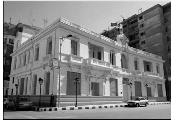
Fig. 2.45 Bank of Alexandria, Al-Gomhuriyya St (former Anglo Bank, then the Italian Bank, then Barclays Bank) © A. Bendary
