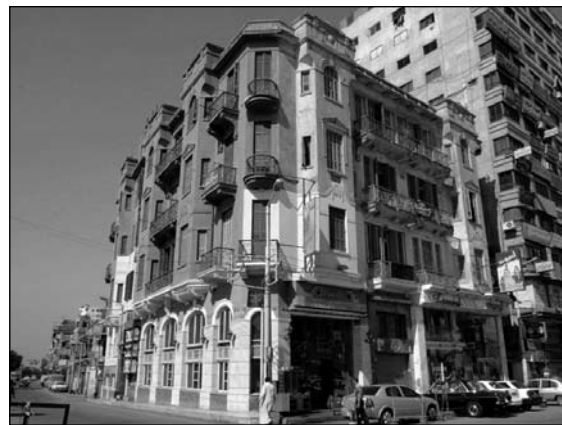
Fig. 2.52 Commercial Residential building, El-Thawra St. © A. Bendary
