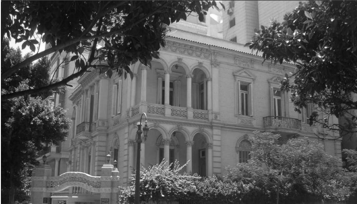
Fig 3.23 Rose El Youssef building, Down-town Cairo © S.Attia
