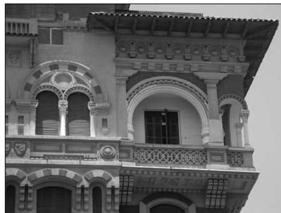
Fig. 3.20 Fine architectural details of buildings © ALEXMed
