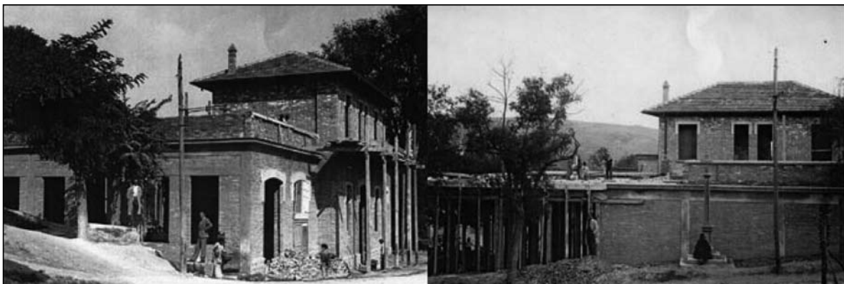
Fig. 3.54 The work-site in 1929. (Historical Archives CMC s.p.a of Ravenna).
