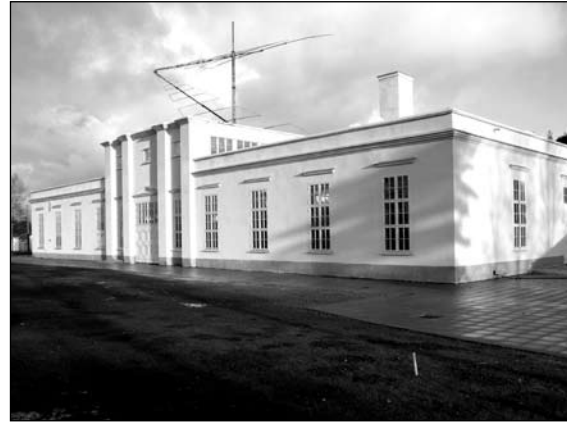
Fig 1.5. Varberg Radio Station © OUR PLACE THE WORLD HERITAGE COLLECTION, www.ourplaceworldheritage.com
